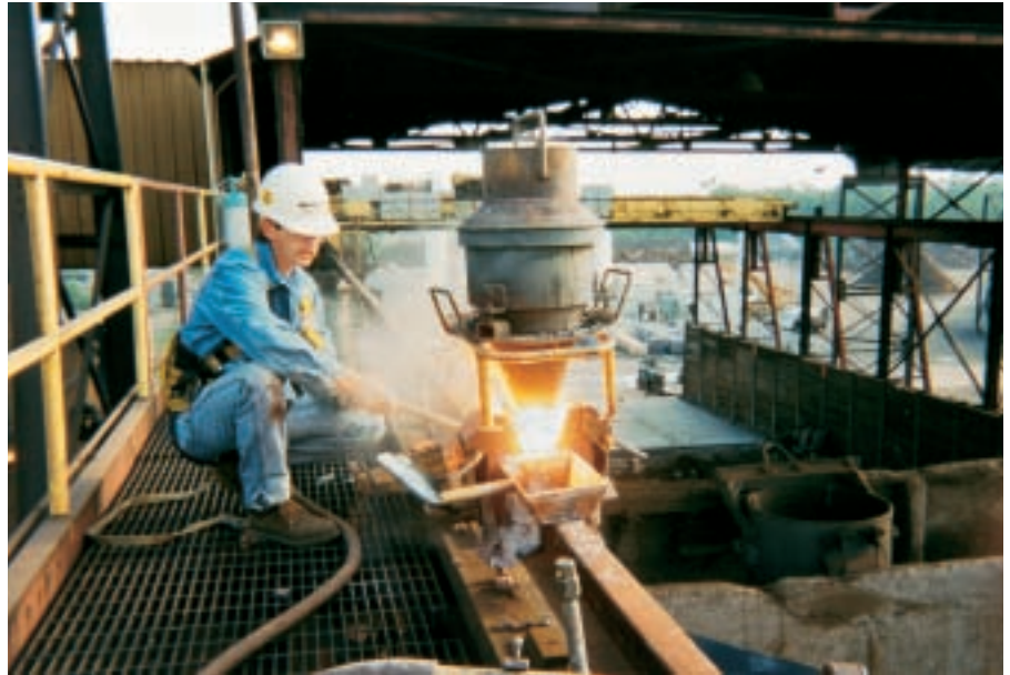
Thermite welding in action.
