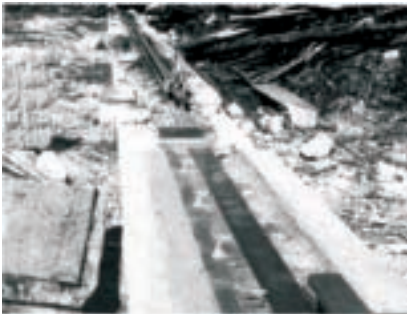
Complete Runway Rebuild
