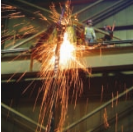
Gantrex Flash-Butt Welding Overhead Rail.
