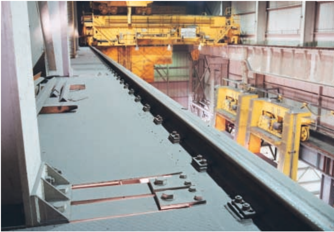
Melt Shop Crane Runway
