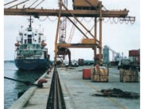
Container Crane ground track
