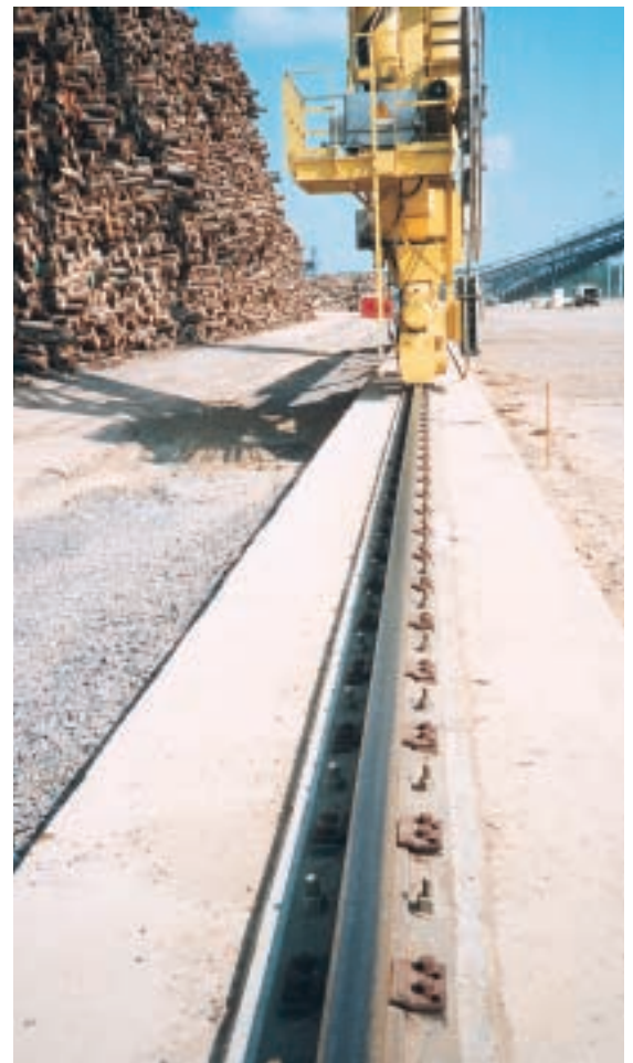
Log Handling Crane Runway
