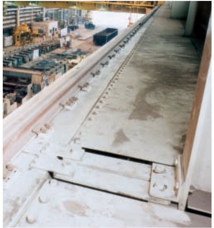
Caster Runout Crane Aisle
