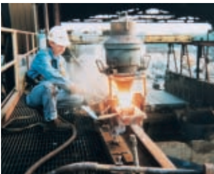
Thermal Rail Welding
