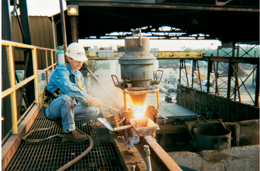
Thermite welding in action
