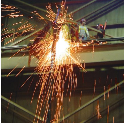
Gantrex Flash-Butt Welding Overhead Rail
